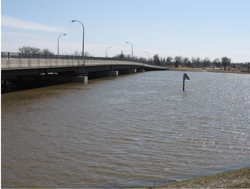
Figure 4. Red Lake River at the Murray Bridge crossing in East Grand Forks
